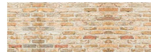
M24 Brick Wall
